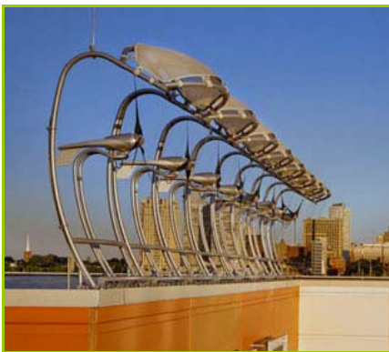
AeroVironment roof parapet turbine
