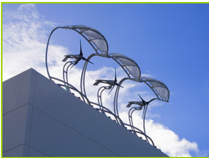
AeroVironment roof parapet turbine
