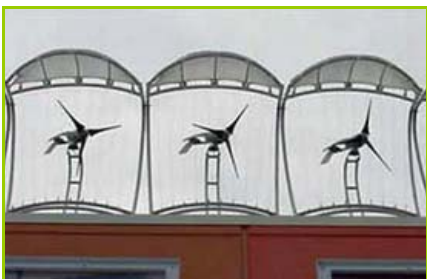
AeroVironment roof parapet turbine
